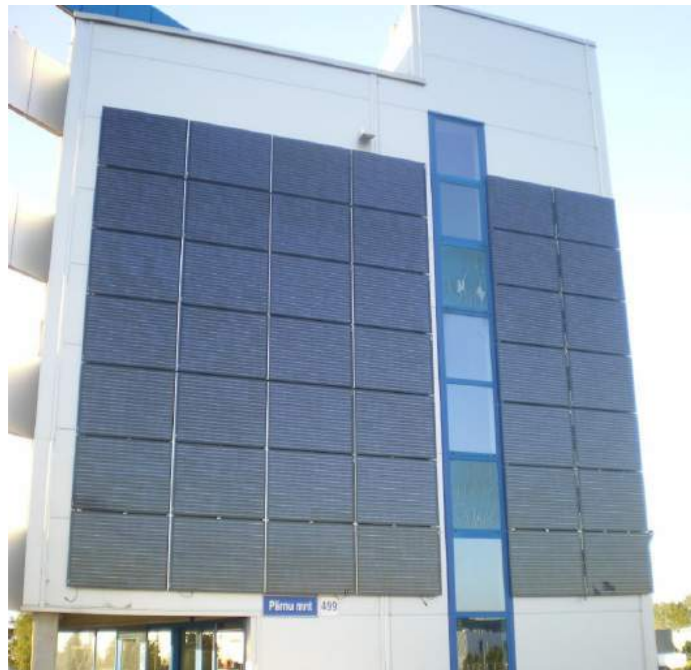
Baltic Disk integrated facade, 12 kW, Estonia
