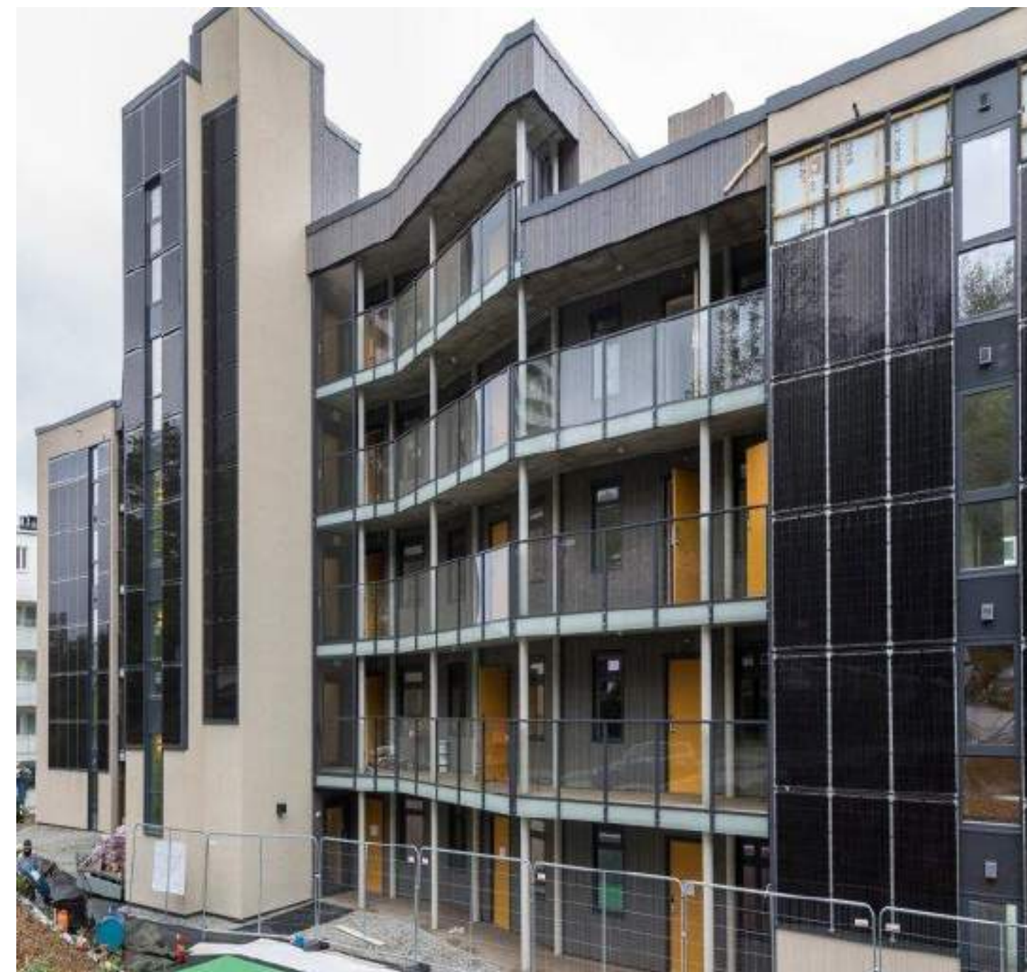
First apartment building BIPV, 42 kW, Norway
